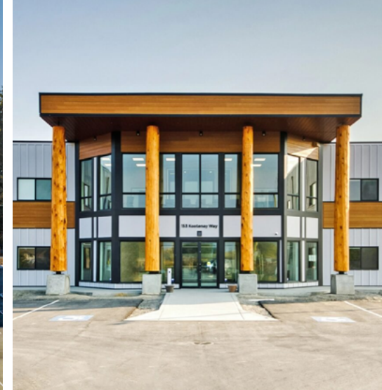
NRB Modular: SCFS Agency Office Building
