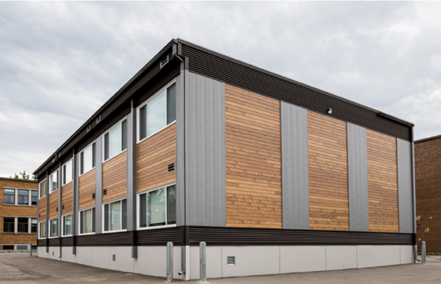
NRB Modular: 4-Storey Multifamily Housing
