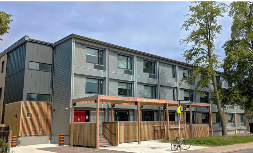
NRB Modular: City of Toronto Supportive Housing
